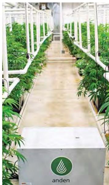
**COMMERCIAL COMPONENTS:** The combination of continuous watering of plants and the sheer physical size of many grow facilities requires dehumidifiers with commercial-grade componentry and capacities, such as this one from Anden.
