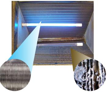
**Example No. 2:** A ten-year old air conditioner coil with a UV bulb placed too close to the end coil. Most of the coil was clean, but the 25% over 8" away grew mold and bacteria actually blocking air flow of 25%. This installation was of some value to the client, but not 100%.
