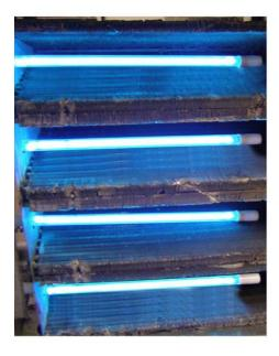
Example No. 4: A large residential coil could require nine UV bulbs to provide good UV protection for mold/bacteria growth. This will add approximately 300 watts of heat energy to the air conditioner system. However, the mold/bacteria protection and subseair flow quent savings would make this installation worthwhile.
