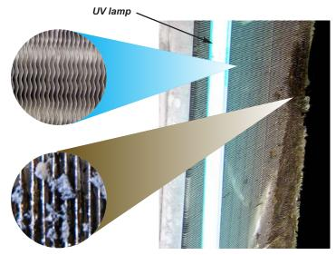
**Example No. 3:** A small air conditioner coil with one UV bulb mounted in the center. Only one-half of this coil has UV protection as the outer sections have no UV bulbs. Exhibit 3 shows how the light does not go through the coil as the geometry of the fins will not permit it.
