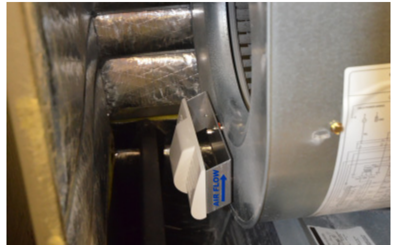
QUAD-DM™ mounted to blower housing
