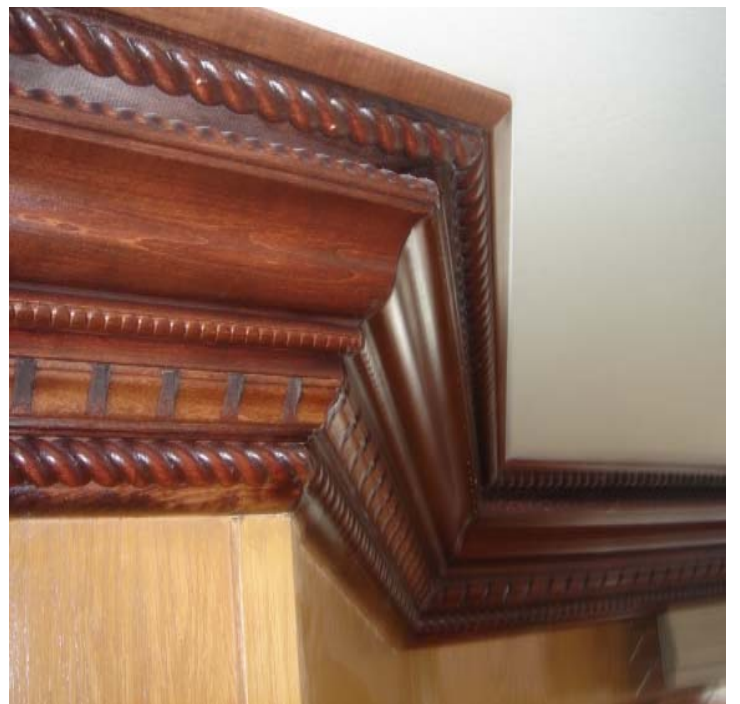
12 piece crown molding with built-in HVAC vent
