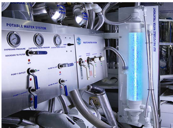
Envision's engine room water treatment system
